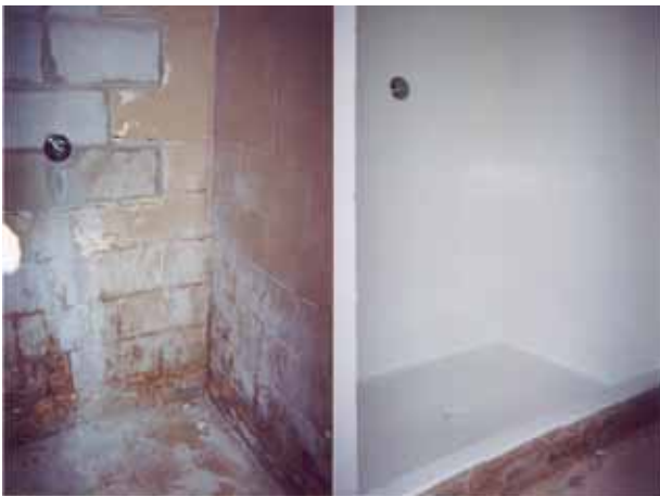
Showers: Before and After
