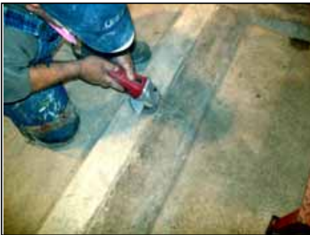
Grinding the Curb
