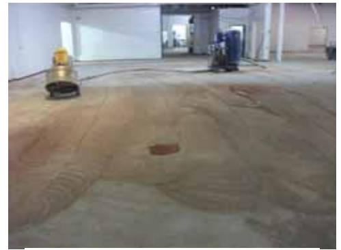
Grinding the Floor
