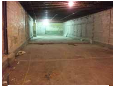
Dry Storage Area
